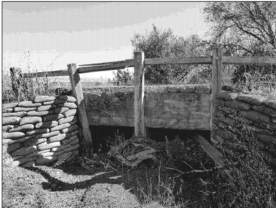
Figure 3.5-5 Tick Creek Branch Culvert
